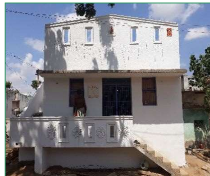
Exhibit 5.6: Subramaniyan Ramalingam (TN2074880), Athanakurichi VP, Mudukulathur Block, Ramanathapuram District Completed inspected on 01/03/2018 01:44:00 hrs
