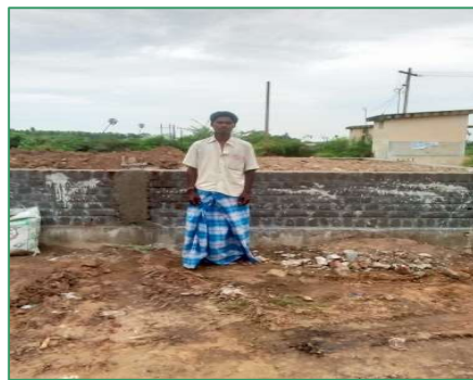
Exhibit 5.5: Smt. Vijaya (TN1180342), Perungalathur, VP, Cheyyar Block Tiruvannamalai District Roof cast inspected on 22/10/2020 at 01:38:00 hrs
