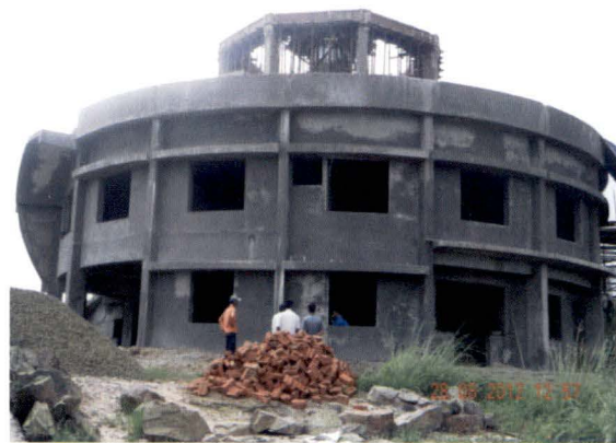
Under construction building for S-Band DWR at Cherrapunji
