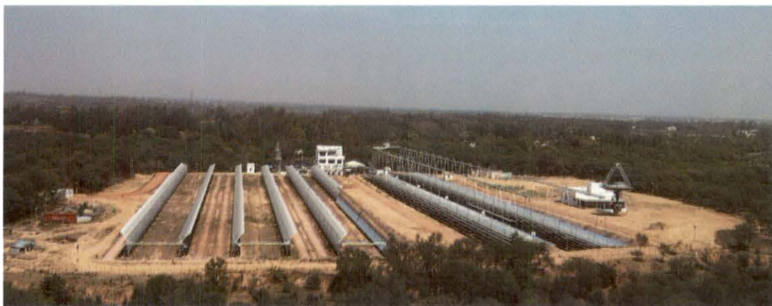
Grid interactive solar thermal power plant developed by IIT under the project
