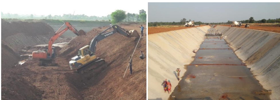
Restoration work of Subarnarekha Main Canal at RD 7.950 km
