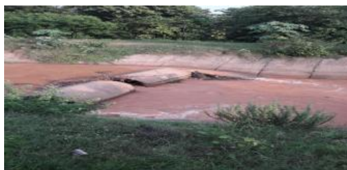
Temporary cross bund in the Golamunda Distributaries at RD2.345 km
