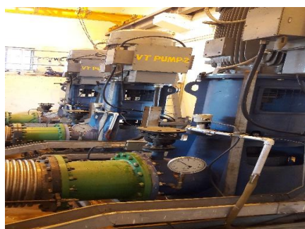
Pump House of Amath Mega Lift Project
