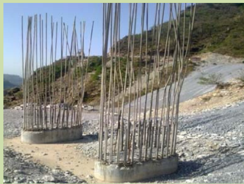
Pier P 19 in dismantled condition
