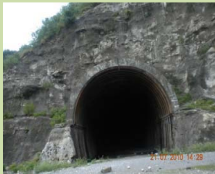
Tunnel T-2 abandoned
