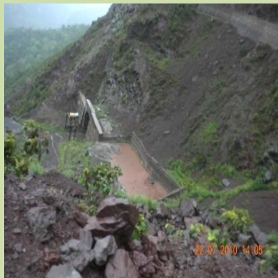
Portal T-6 P2, which was abandoned
