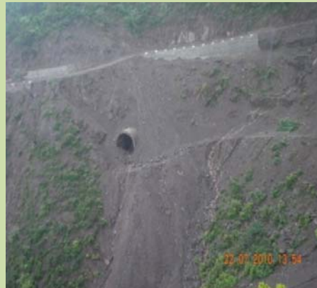
Portal T-8 P1, which was abandoned
