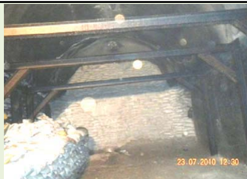
Face of demolished T1 blocked with gunny bags
