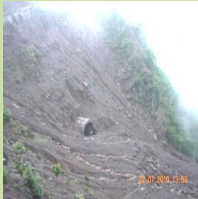
Portal T-7 P2, which was abandoned
