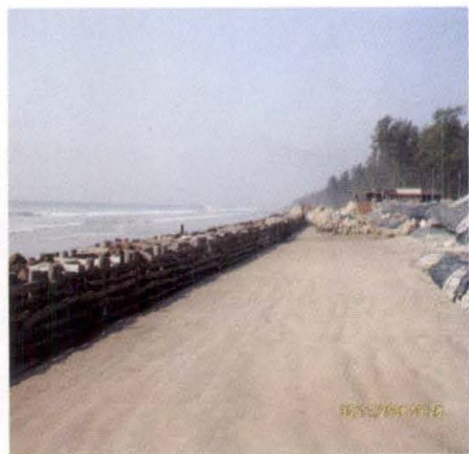
Boulder protection work to protect Geotubes
