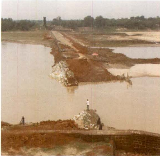
Breached low weir of Anicut after the flood of July 2008
