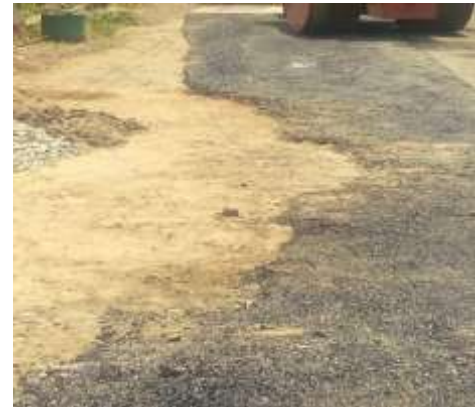
Picture 3: New bituminous layer laid on non-bituminous surface without clearing the loose soil and applying prime coat for bonding caused peeling off of the new layer (photo taken on 14/09/2018)
