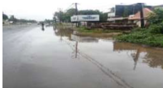
Picture 9: Lack of side drain caused water logging preventing access to bus waiting shed in NH 66
