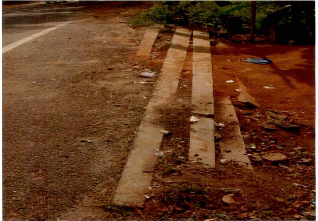
Poles stacked on way side and buried under soil and bitumen at Thodupuzha EC.
