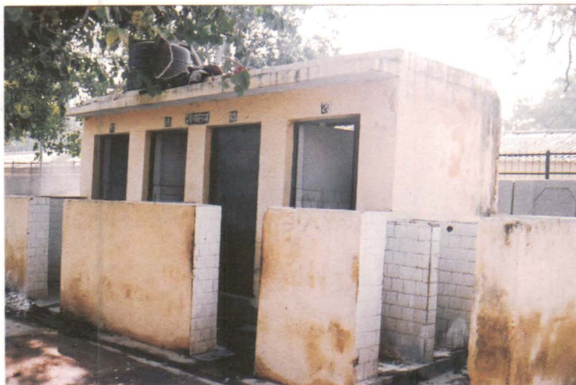
Figure – 4: A toilet block in a primary school, Khichripur
