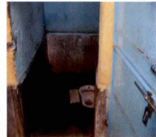
Toilet at Jaipur
