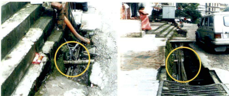
Pipelines running through drain in Tibet Road area
