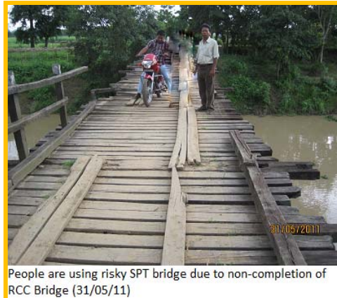
Incomplete RCC Bridge at Hayangaon (31/05/11)
