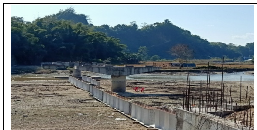
Bridge over Pachin river as on Dec 2019
