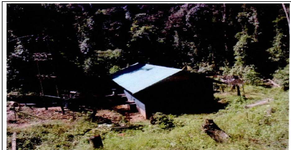
Power House lying idle
