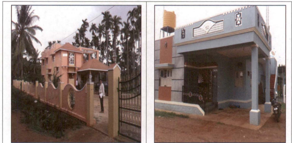
Photographs showing the houses where BPL status was doubtful (GPs, Annehal-07.08.2014 and Alagawadi-04.04.2014 of ZP, Chitradurga)
