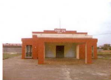
Renovation of Town Hall, Subarnapur
