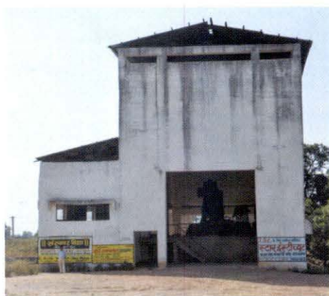
Incomplete SHP at Tejpura
