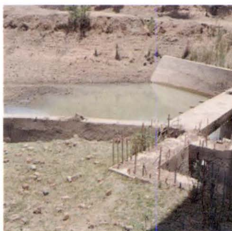
Incomplete SHP at Paharma
