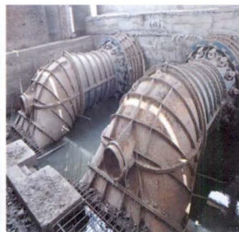
Draft tube with elbow section at Paharma SHP
