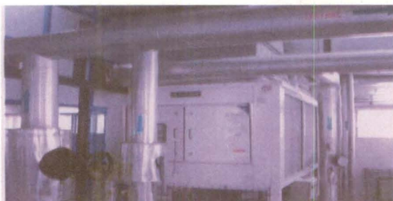
Clean room facility constructed under RAIF
