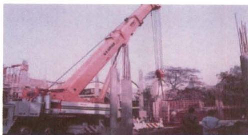
Civil Construction under progress under IFRT
