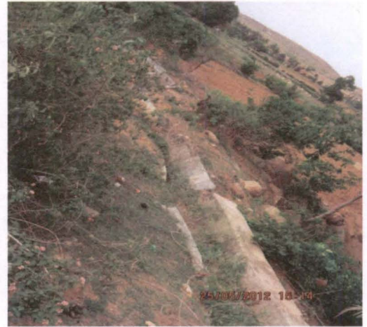
Photograph 3: Canal repair work executed by GP, Tirumani (25 May 2012)
