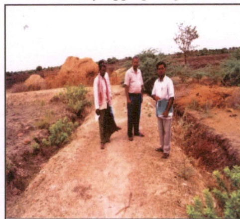
Photograph 4: Execution of mud road in Devdurga taluk, Raichur district (12 June 2012)
