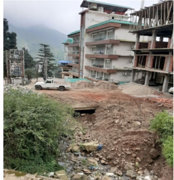
Covered nallah on Government land (Bhagsunag to Dharamkot road) (21.09.2019)
