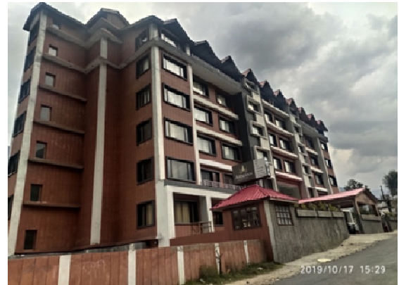
Shuru area (in Manali Agglomeration) having multi-storeyed commercial buildings (17.10.2019)
