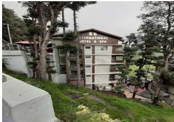
Building with no. of storeys exceeding permissible limits in Dalhousie (03.10.2019)
