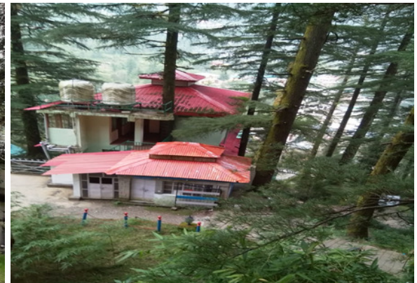
Tree covered within building in Dharamshala (21.09.2019)
