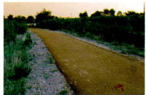
Two km chainage on Mangalapur-Bhimakunda road where there is no nullah
