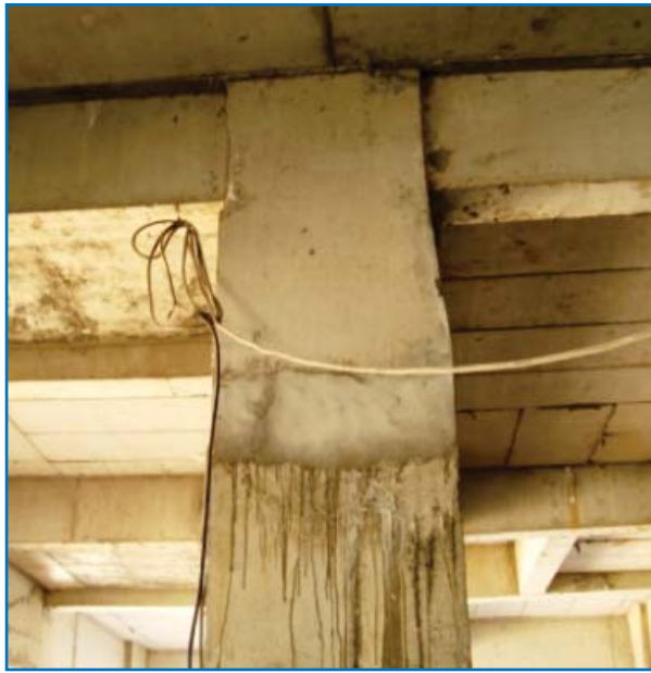
Tower -10: Tapered column (LB) Report No. 9
