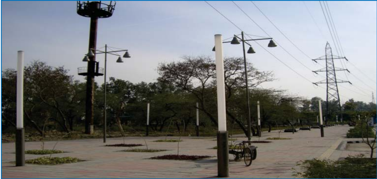
Fittings worth over Rs. 50 lakh installed opposite IG Stadium
