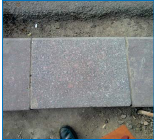
Granite kerb fixed at work site
