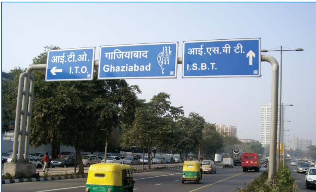
Cantilever mounted signage
