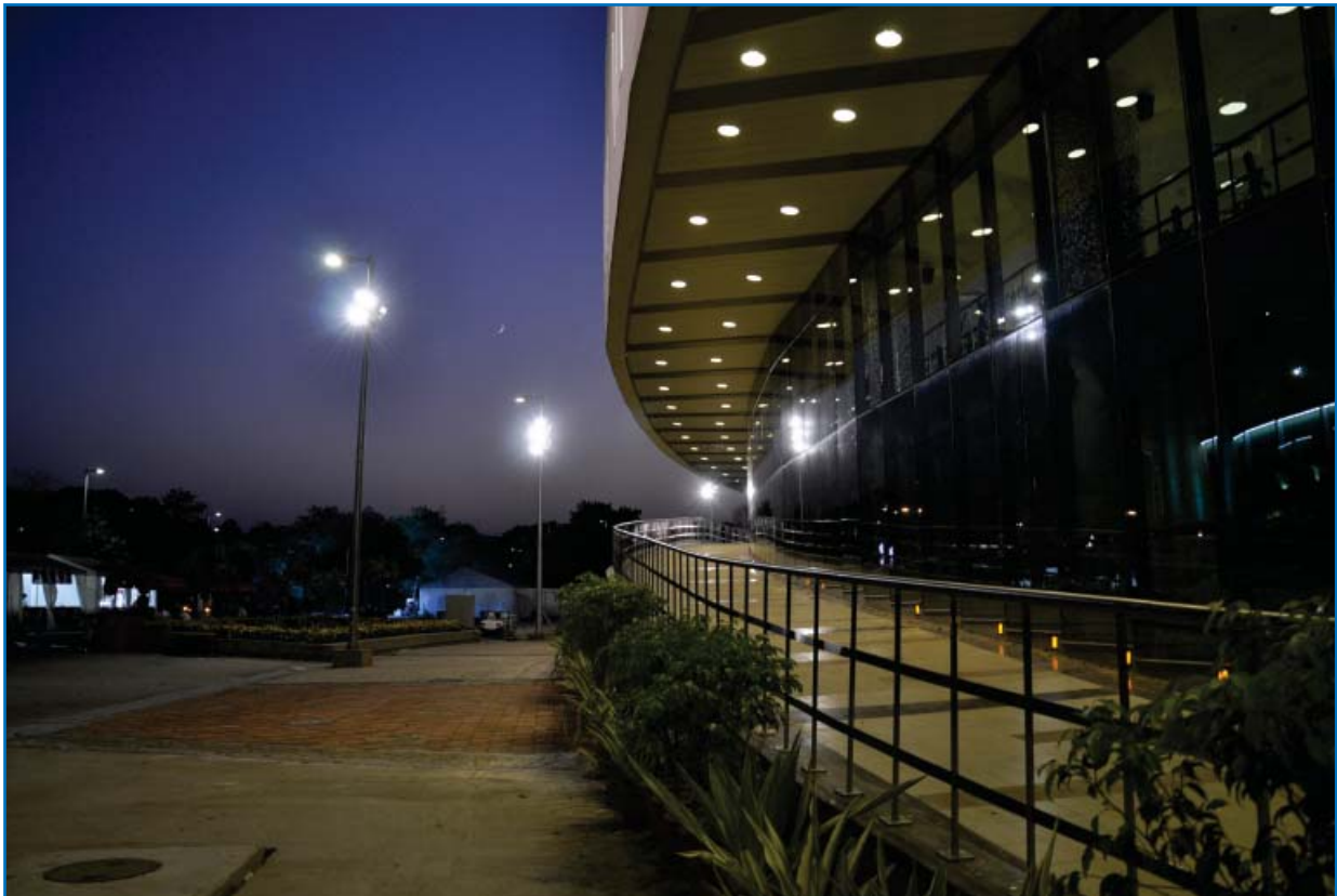
IG Wrestling Stadium
