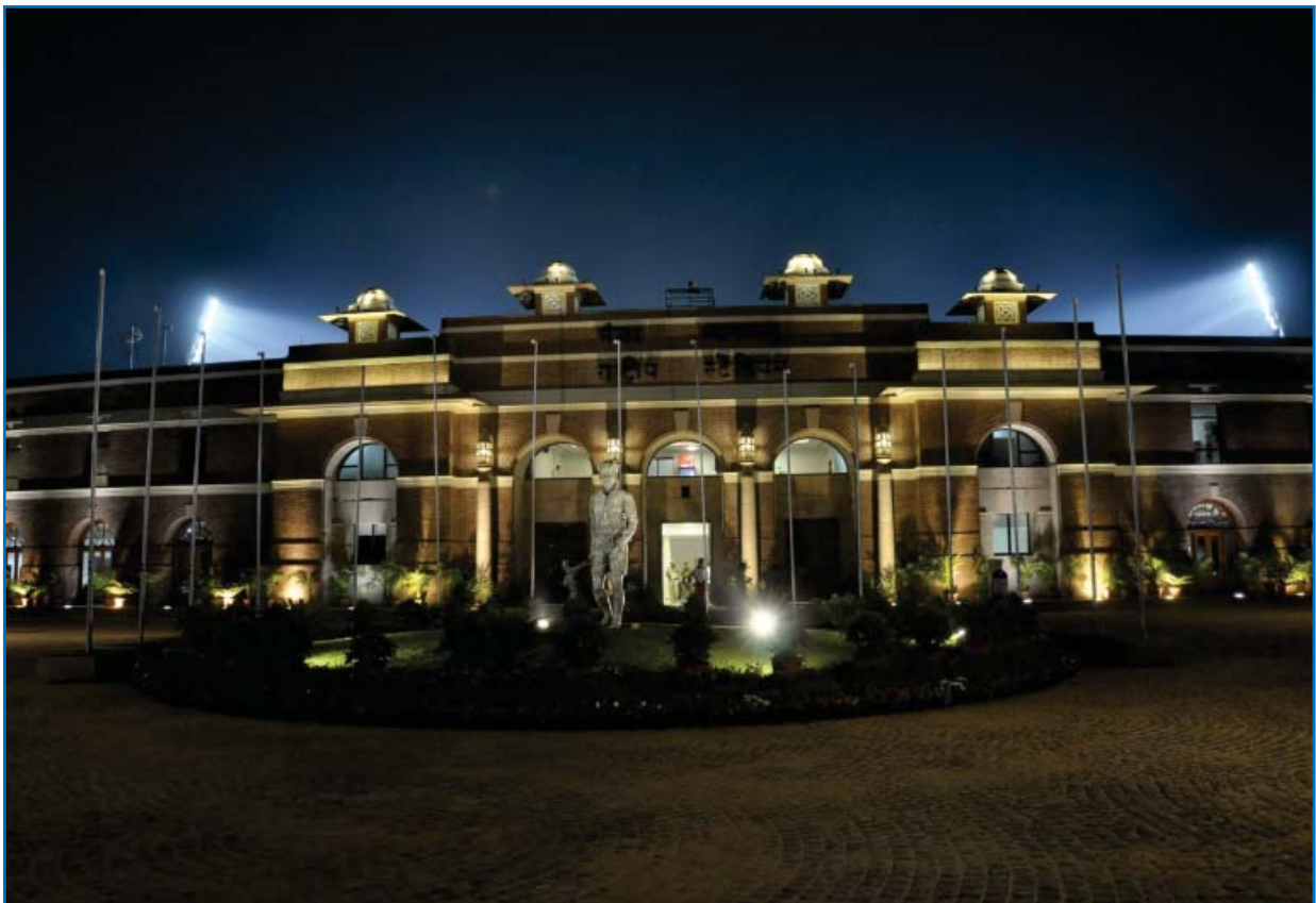
MDC National Stadium
