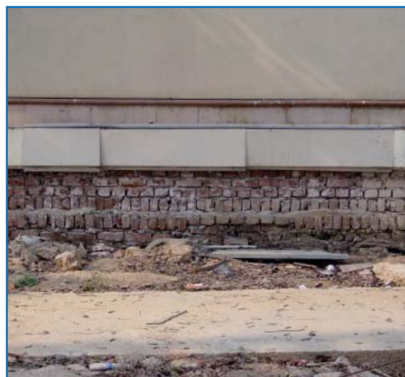
Unplastered Wall of JNS
