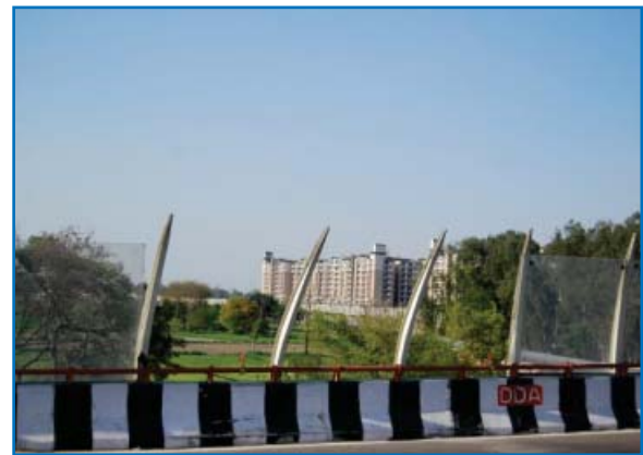
Noise barrier on NH-24
