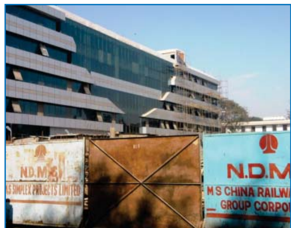
Barricading in the names of main/sub-contractor at worksite
