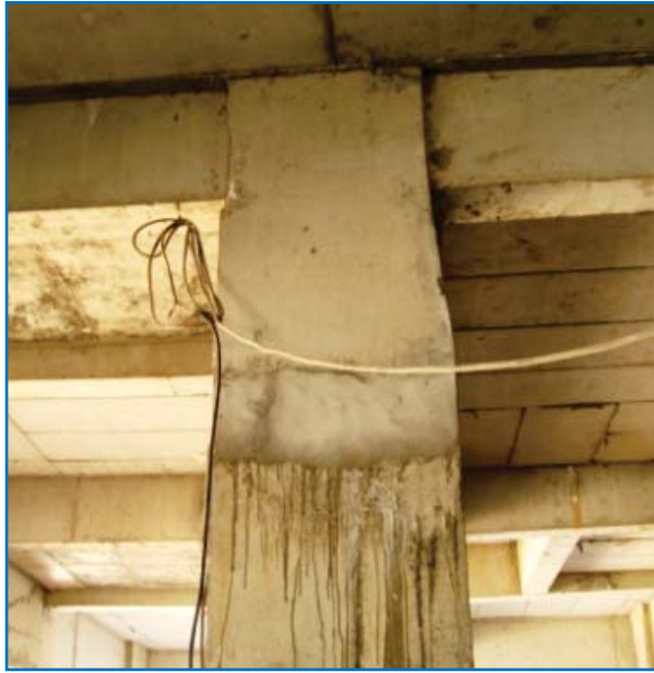
Tower -10: Tapered column (LB) Report No. 9
