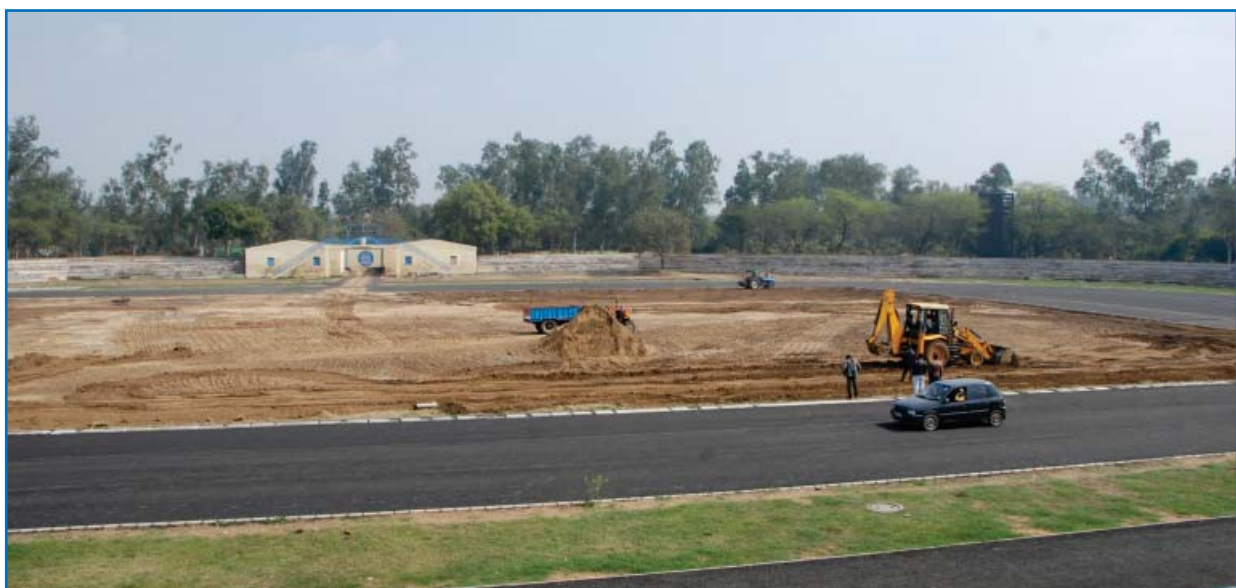
Construction site of Training Facilities at CRPF Campus, Jharoda Kalan
