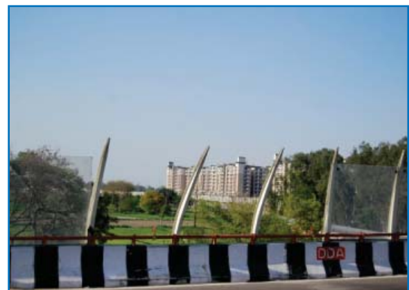
Noise barrier on NH-24
