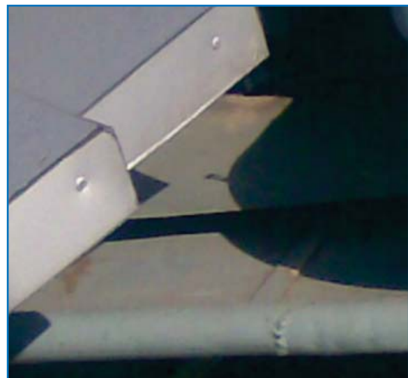
Riveting of ACM to frame
