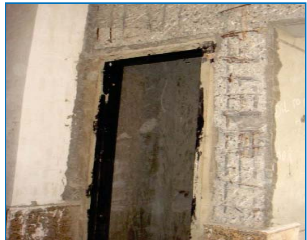
Chipping and cutting of reinforcing steel – Report No. 11
