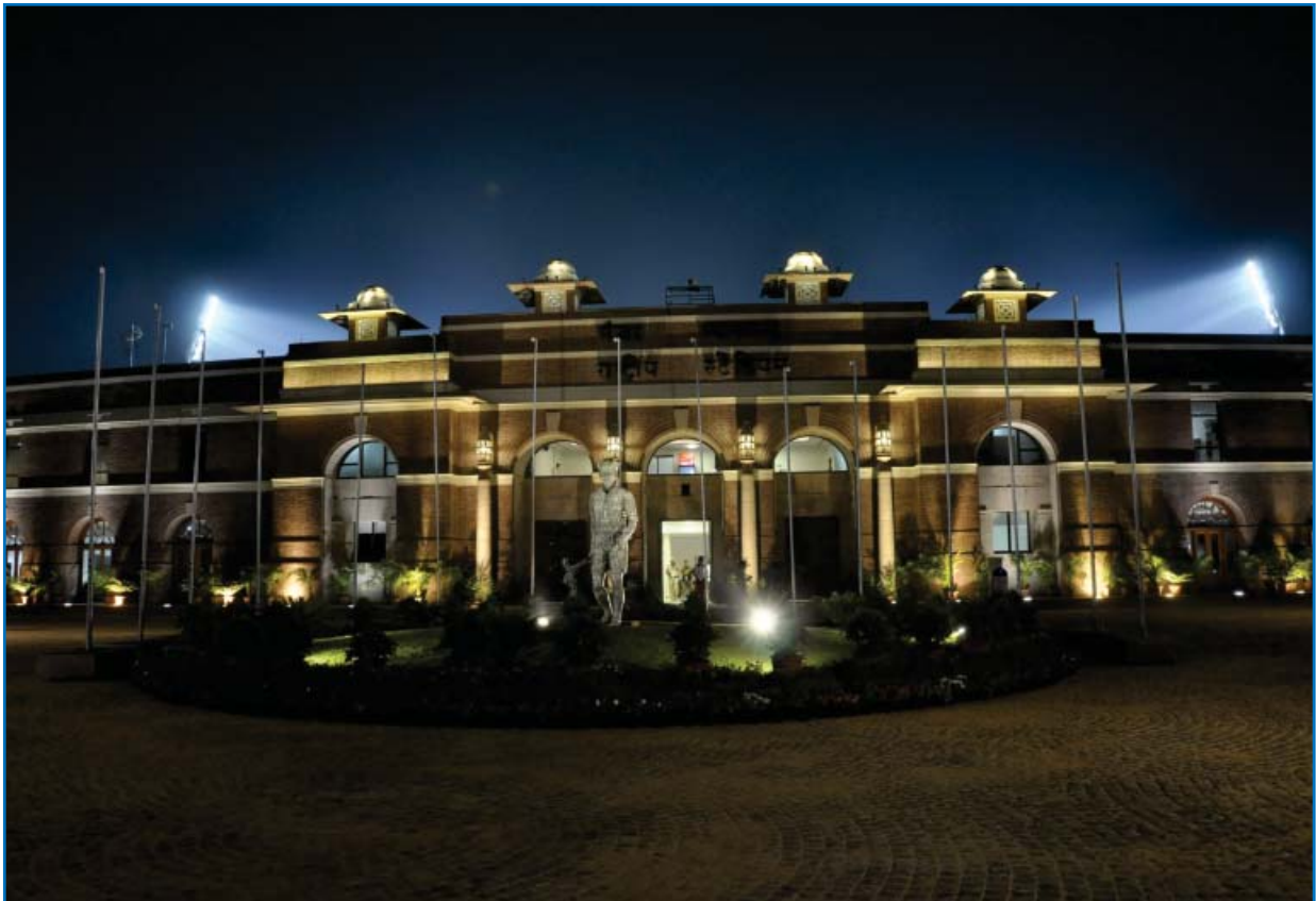
MDC National Stadium
