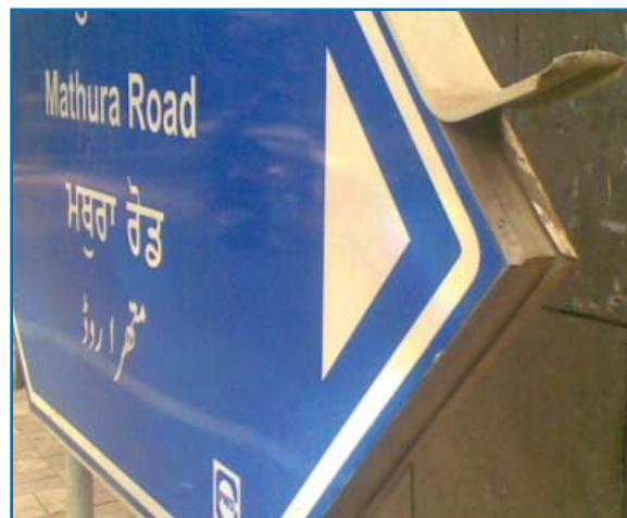
Aluminium Trim peeling off from frame
