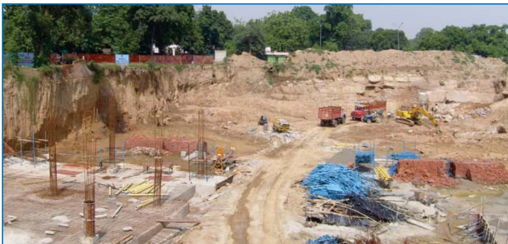
Picture of the construction site at Talkatora Indoor stadium indicating space available for construction activity.
