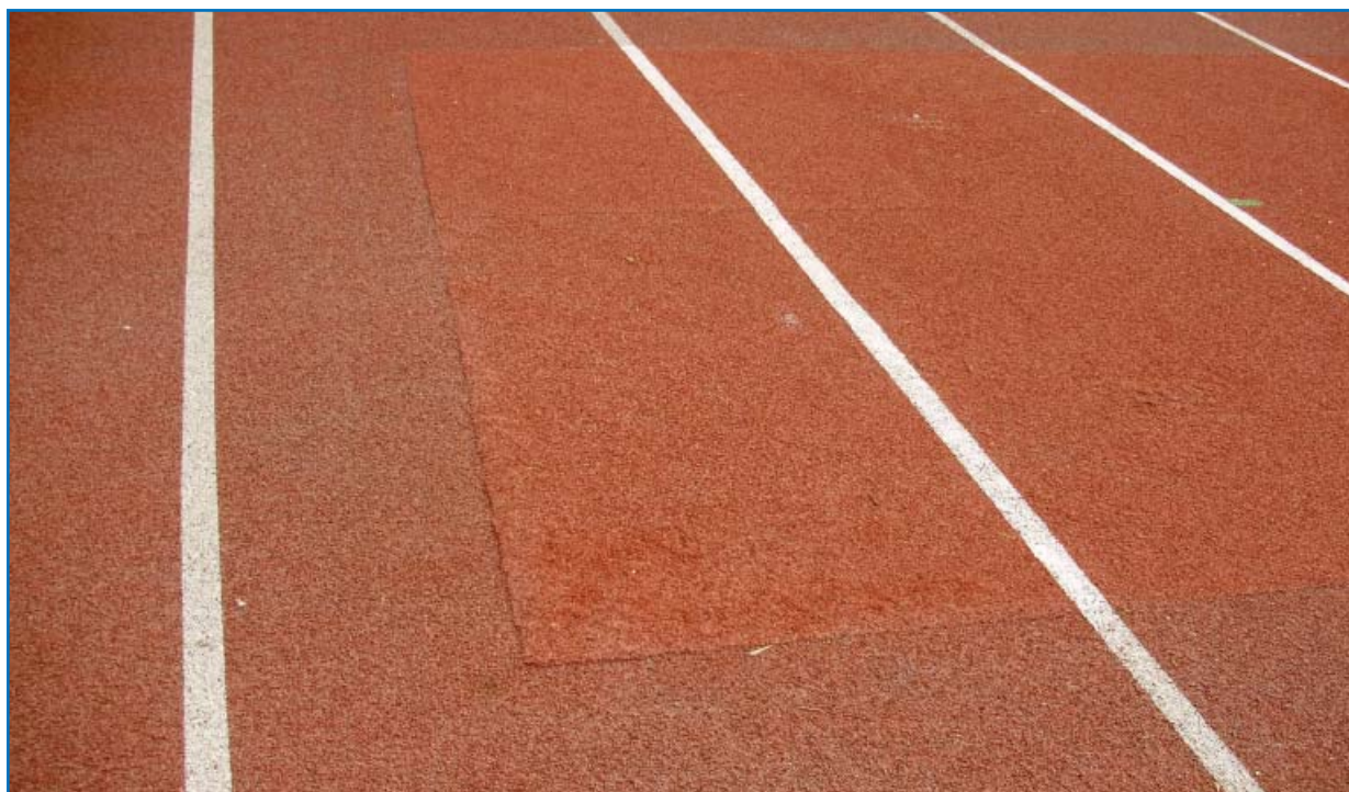
Patch work on the athletic synthetic surface track
