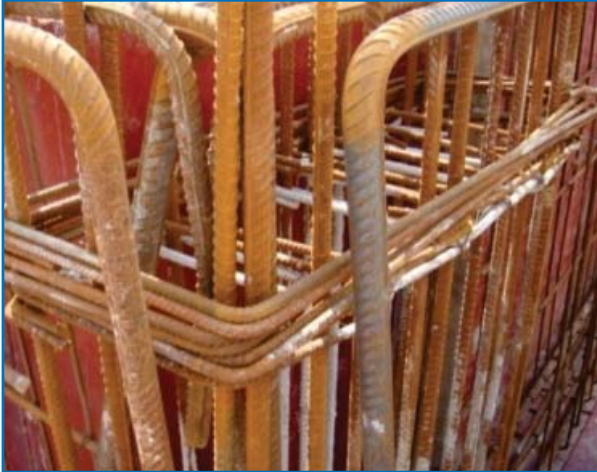
Main bars of the beams located outside the vertical bars of the column - Report No. 3
