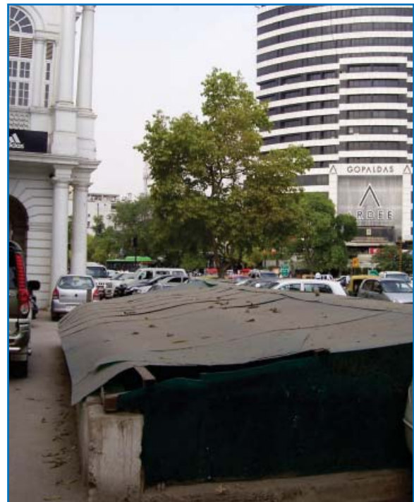
Covered subway entrance after re-filling
