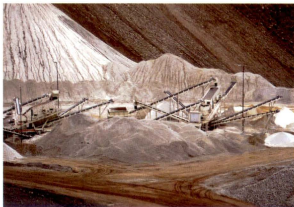
Srinagar hydro project: Stone crusher
