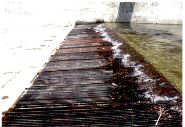
Loharkhet : Trench type weir
