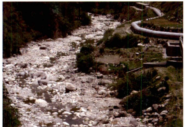
Debal - Downstream flow; Penstock is seen parallel
