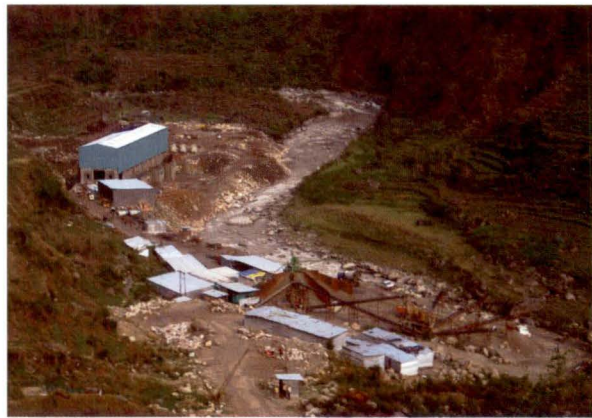
Bhilangana-III : Stone crusher
