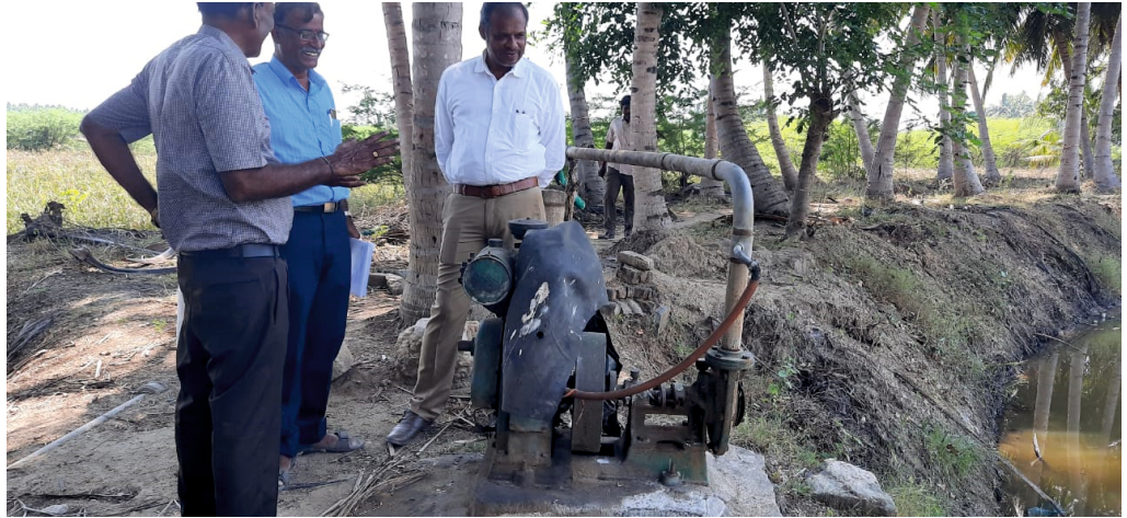
Figure 2: Illegal drawal of water in Pallapalayam Left bank channel
