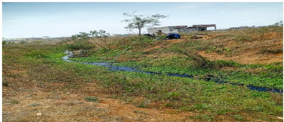
Figure 6: Siltation with bushes in the lined channel
