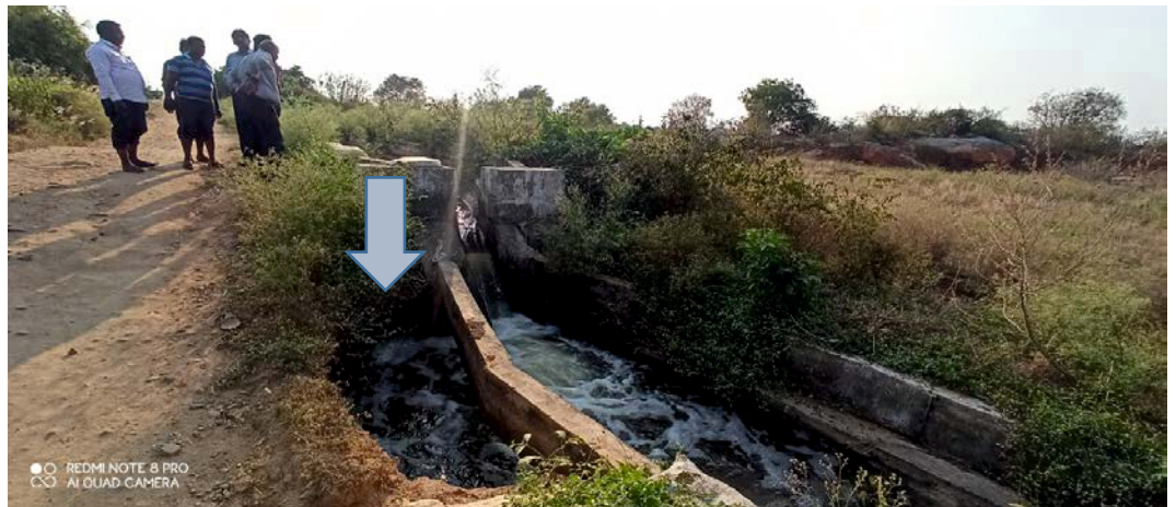
Figure 6: Siltation with bushes in the lined channel
