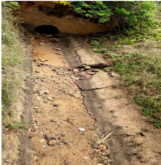
Figure 4: Damages in the outlet channel
