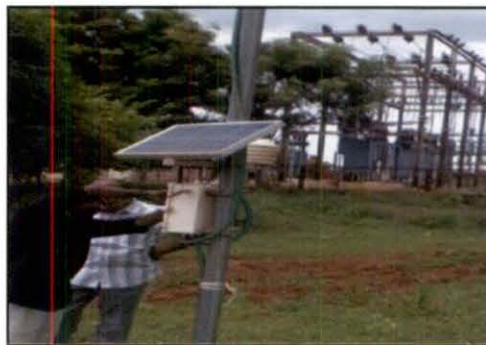
AWS (11724), Dumpalgattu, Kajipet Mandal, Kadapa district (Andhra Pradesh) located near Dumpalgattu electric substation
