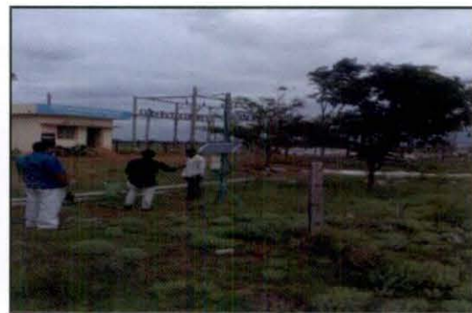
AWS (11717), Ramapur, Duvvur Mandal, Kadapa district (Andhra Pradesh) located near Chintakunta electric substation
