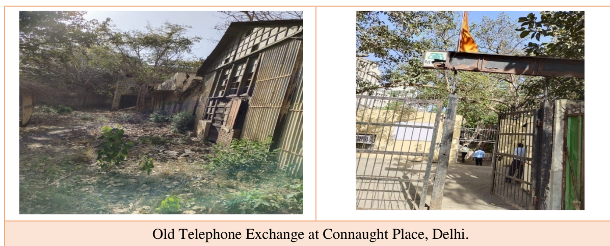
Figure 5.1: Old Telephone Exchange building at Connaught Place, Delhi
