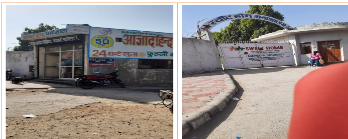
Illegal encroachment of MTNL properties at Najafgarh Gaon Sabha, Delhi
