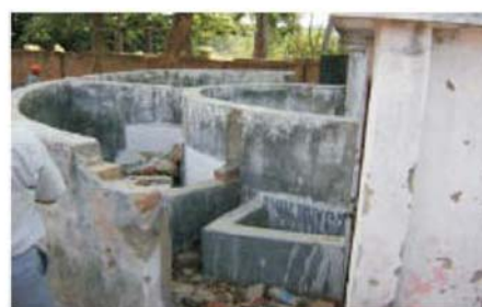
Middle School, Khajuri, Simri Bakhtiyarpur, Saharsa, Period of construction : 2008-09
