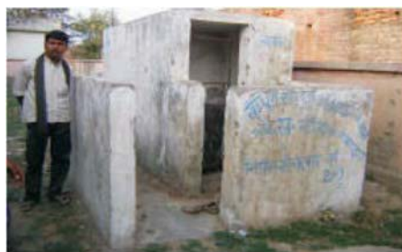
Middle School, Darbeshpur Dakshini, Patna, period of construction : 2007-08
