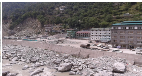
FPW at Chamoli (After Reconstruction)
