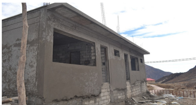
Under Construction Buildings for Tirth Purohits by NIM
