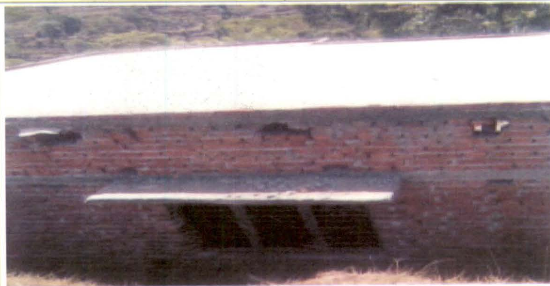
Incomplete Government Primary School Kas, Thudi
