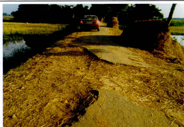
Picture showing broken road in the work 'Improvement i/c MBT of a road from AMPT road to Haribanga village via Bholarbita (0.300 Km) under RIDF-XX' which was completed during February 2017. Date of joint physical verification: 05.06.2018
