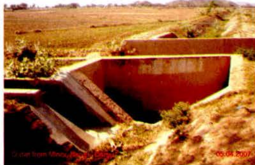
Dry outlet for water works at Nangal Dargu
