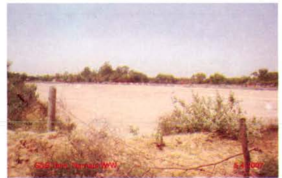
Empty storage and sedimentation tank at Narnaul water works
