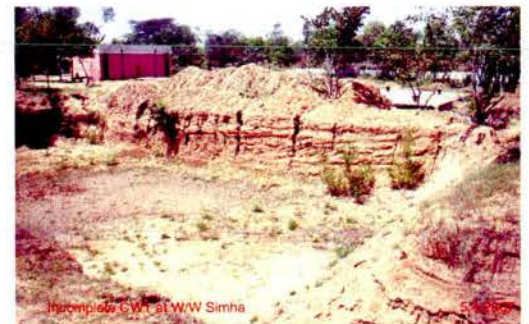
Incomplete second clear water tank at water works Seehma
