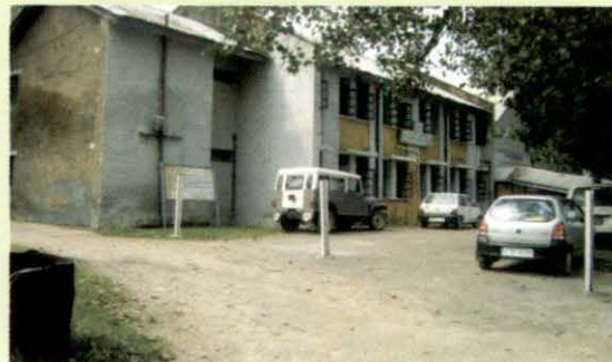
Primary Health Centre Bhota without boundary wall
