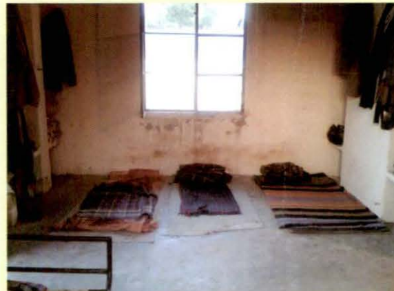
Rest room for males at PS Amb without any basic facilities like attached toilets, baths, cots, bedding, etc.
