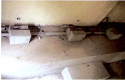
Installed pump sets removed from platform
