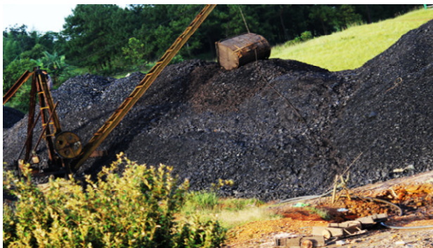
A mining site at Dkiah, Khliehriat. Powered crane can be seen indicating that fresh coal mining is taking place
