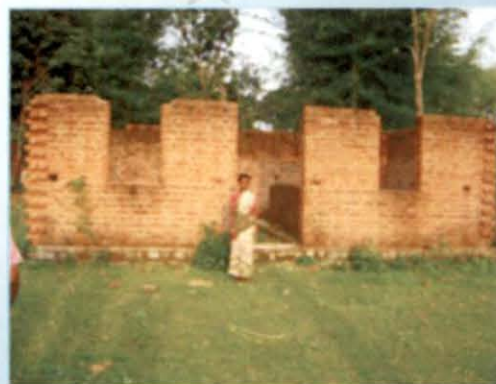
Picture-6: IAY house in scheme no. 198/08-09 at Sodag GP in Namkum block of Ranchi district and ₹ 35,000 (final payment) was paid to beneficiary.
