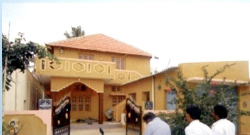
IAY house in Manchanayakanahalli GP, Ramanagara TP, Ramanagara ZP
