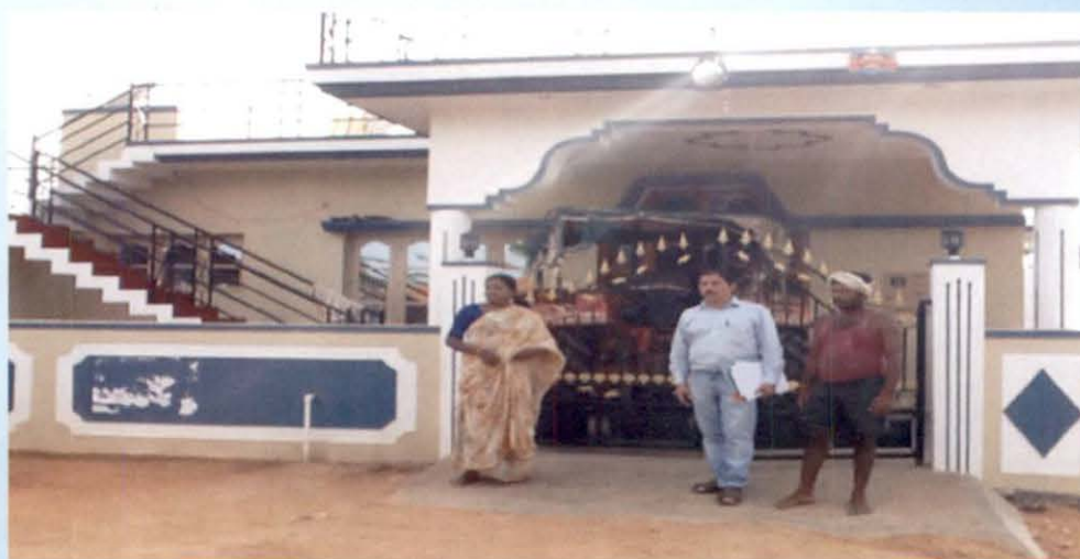
IAY house in Hebbadi Village, Melapura GP, SR Pattana TP, Mandya ZP
