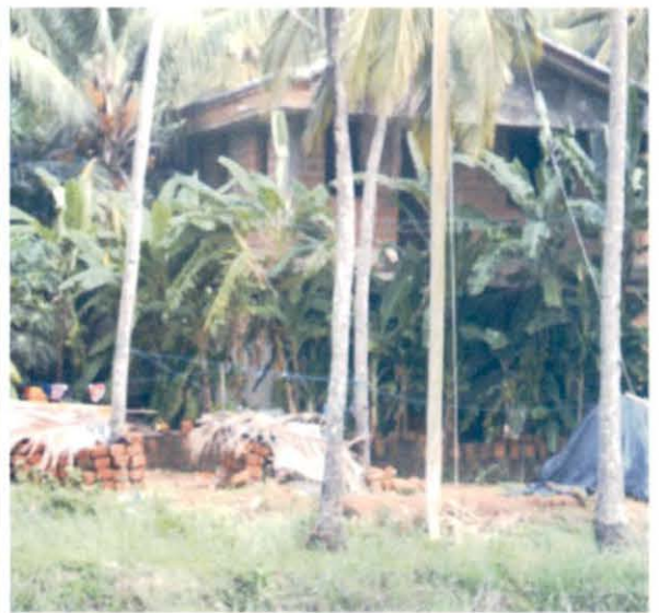
New House under construction of Mrs. 'Y'
