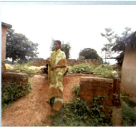
IAY house in scheme No. 67/2009-10 at Pali GP in Ratu block of Ranchi district abandoned after ₹ 35,000 (final payment) was paid to the beneficiary.
