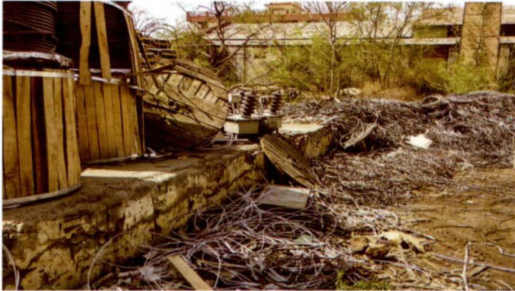
New cables and scrapped conductor lying at JPDC ACOS
