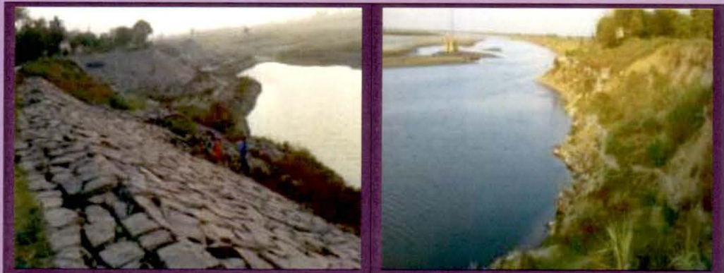
Anti-erosion works were executed between km 7.100 and 7.500 on Bokta Barwar embankment in Gorakhpur district during 2012-13 (left) without assessing the effects of the construction on other sites. Subsequent to the works, the river Rapti hit the embankment between km 7.505 and 7.550 (right), which led to flood fighting works in 2013-14 (Dated: 28.04.2014).
