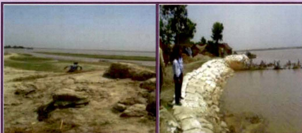
Incomplete Sharda Nagar to Aira Bridge embankment in Lakhimpur kheri (left) led to river water entering in villages and necessitated anti-erosion works (right) to protect them (Dated: 23.6.2014).
