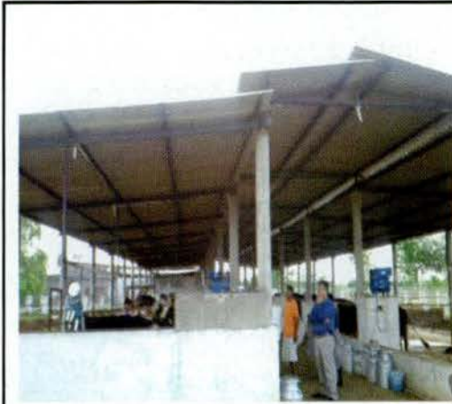
High Tech Dairy Shed at Sherpur, District Ambala constructed as per specifications and design.
