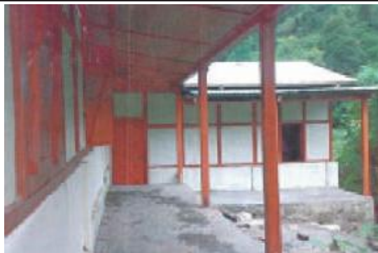
RESIDENTIAL BLDG. FOR 50 BOARDERS AT GOVT. M.E. SCHOOL BOA SIMLA – RAGA Block
