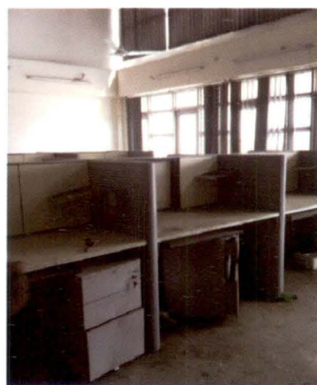
Unutilised rooms in Palika Bhawan
