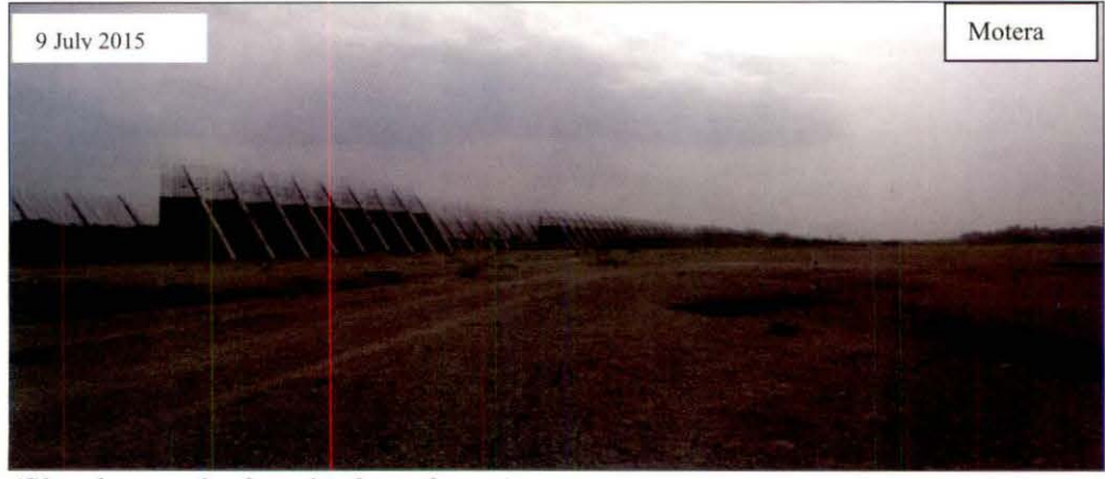
(Showing works done in three depots)
