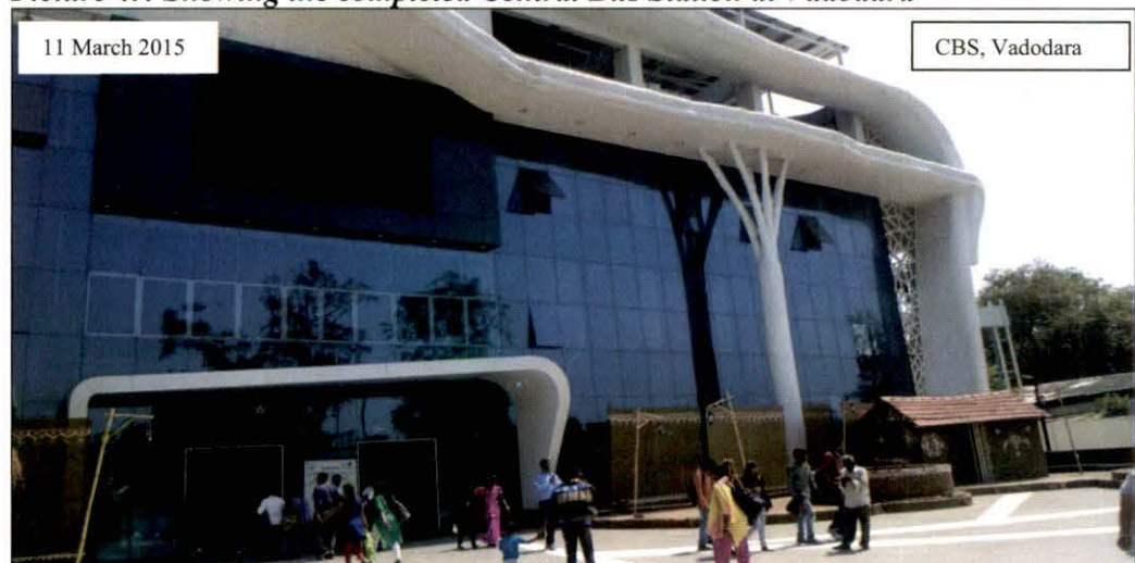
Picture 4.4 Showing the completed Central Bus Station at Vadodara
