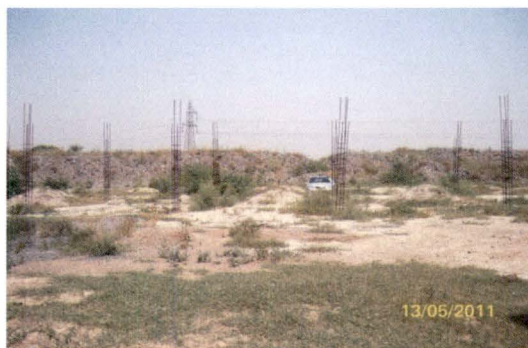
Abandoned old site of SWM Project at Jind Road , Rohtak
