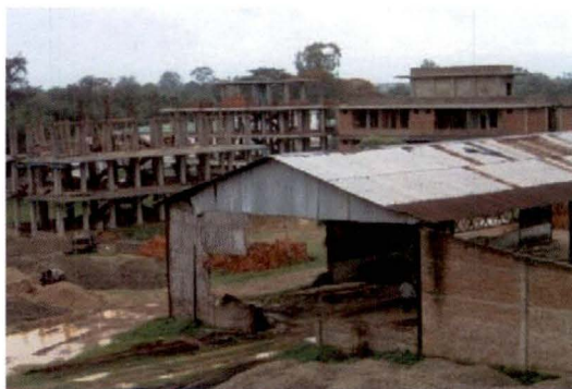
Saw-mill at Burma Camp project site – IHSDP project in Dimapur, Nagaland
