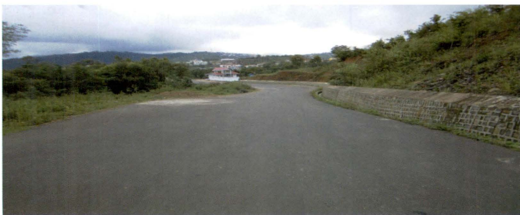
Photograph No. 7.13 of Thizama Road (Refer Para 7.6.4)
