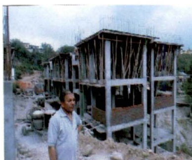
Block Nos. 1 to 6 of IHSDP project in Hamirpur, Himachal Pradesh under construction (18 May 2011)
