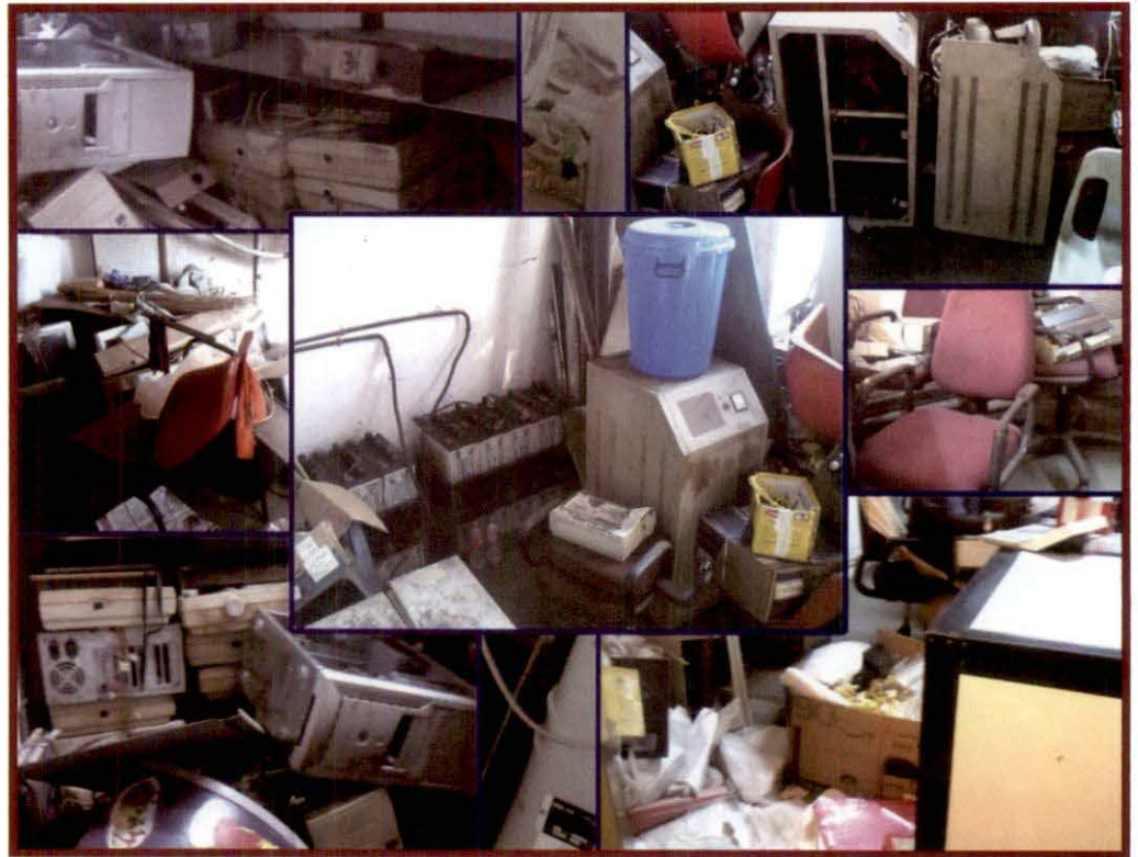
Picture shows dumping of scrap over the UPS, battery and near the counters in Thiruvananthapuram and Malappuram Centres.
