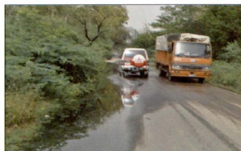
Sewer water flowing on the road at Mirzapur STP on Tigoan road, Faridabad
