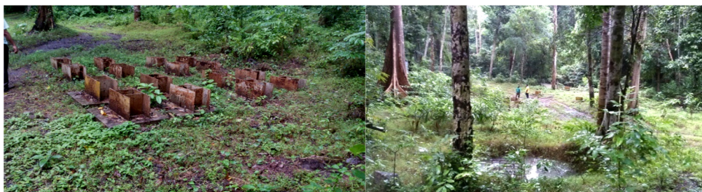
The present status of construction of CW at Chidiyatapu Biological Park
