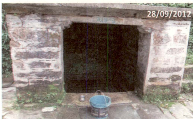
Traditional Naulas have been renovated
