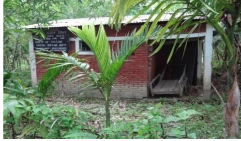
Abandoned Chalchali Dadara Chowk 18 no. AWC under Barhampur ICDS Project, Nagaon (12.06.2014)
