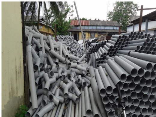
PVC pipe Goalpara lying in open air (18 July 2014)
