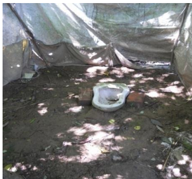
Toilet without sub-structure at Gakhirvety GP, Tinsukia (27 August 2014)
