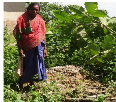
Defunct toilet at Bheluguri GP, Nagaon (8 August 2014)
