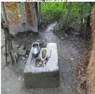
Incomplete toilet without pit at Hatbor GP, Nagaon (6 August 2014)
