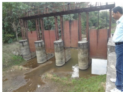
Construction of Head Work (4 March 2014)
