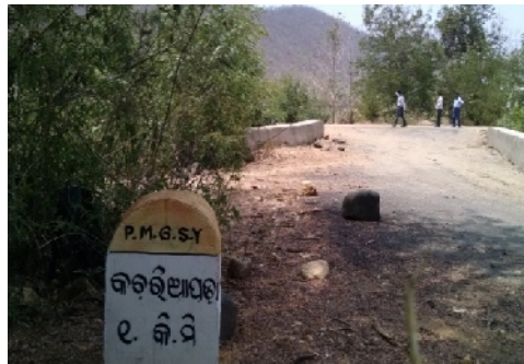
PWD road to Kacheripada ends without construction of 1.000 Km due to want of forest clearance
