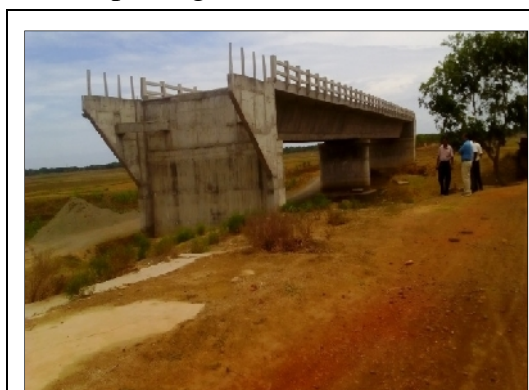
Bridge without approach under RW Division, Kendrapara
