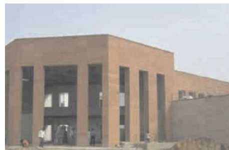
iCED building under construction
