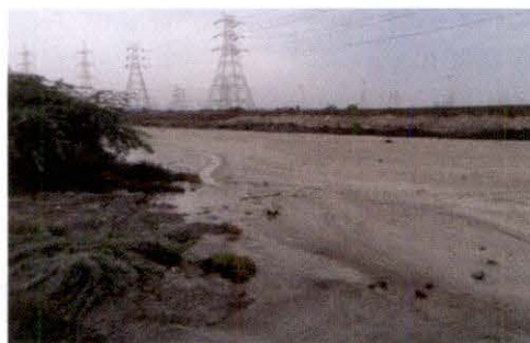
Figure 3- Ash mixed water from NCTPS being led into the Ennore creek
