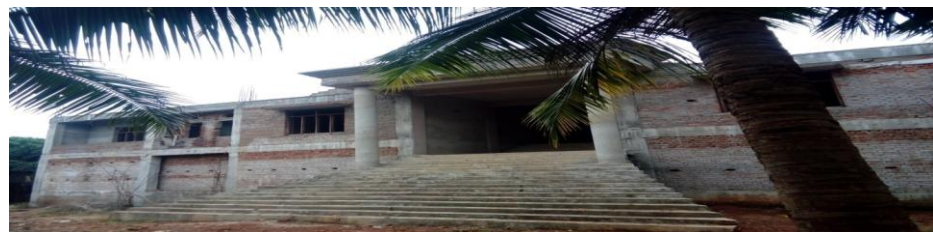
Photograph of incomplete civil defence training institute at Bhubaneswar
